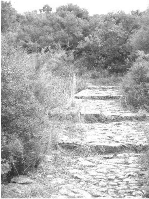
A typical section of kalderimi
